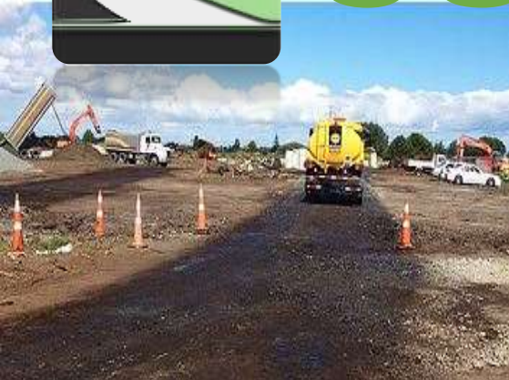
Dust Capping on construction sites
